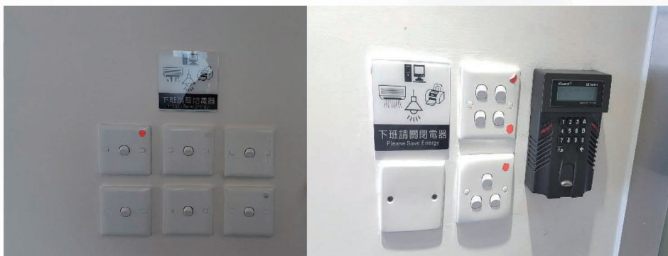
Labels reminding our staff to switch off appliances before leaving the office
