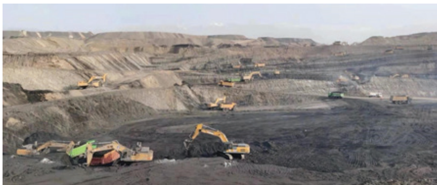
Excavation and separation works by the construction team
