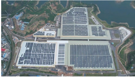
均州工廠三期光伏屋頂俯瞰圖 Aerial View of Phase III Rooftop Photovoltaic Power Generation System of Junzhou Factory
