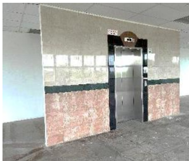
Passenger Lift Lobby
