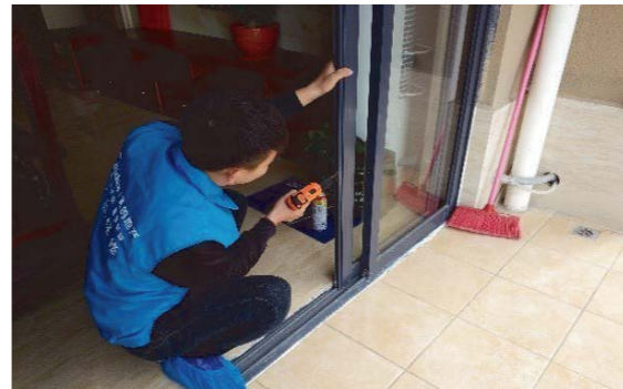
▷ Door-to-Door Maintenance during Beautiful Home Campaign
