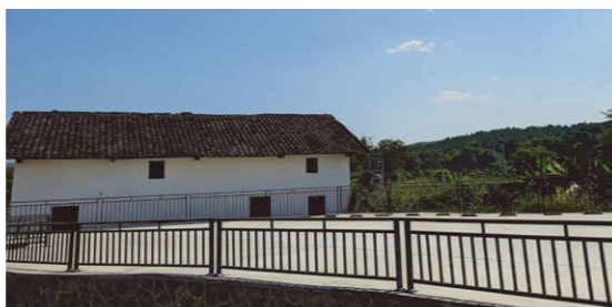
▷ Parking Lot after Renovation
