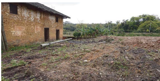
▷ Parking Lot before Renovation
