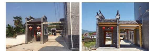
▷ Archway before Renovation
