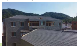
▷ In September 2019, the external facades of 24 houses in Xinwuzu, Jiawon was completed.
