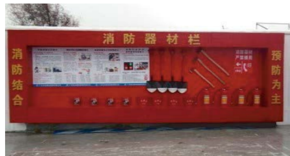
▷ Firefighting Equipment Bulletin Board
