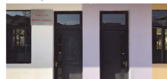
▷ Primary School after Renovation
