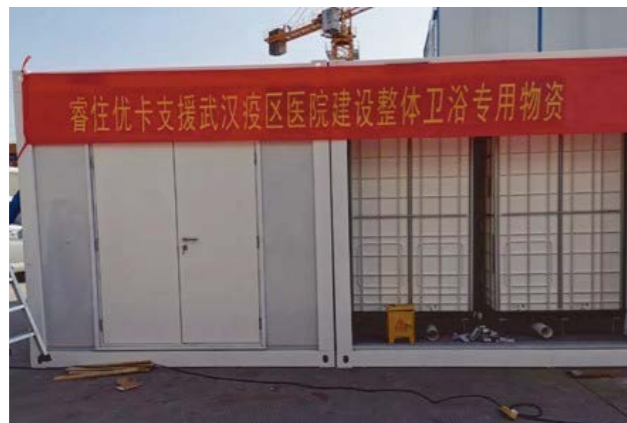
▷ On 28 January, Ruizhu Youka supported the construction of "Xiaotangshan" Hospital.
