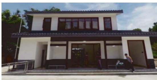
▷ Cultural Activity Room after Renovation
