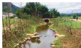
▷ In July 2019, the Dajing River Course Renovation Project of Hefu Village was completed.
