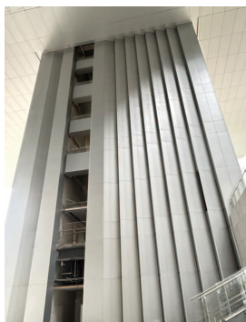
Aluminum curtain wall
