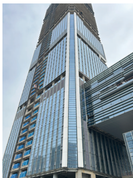
Glass curtain wall
