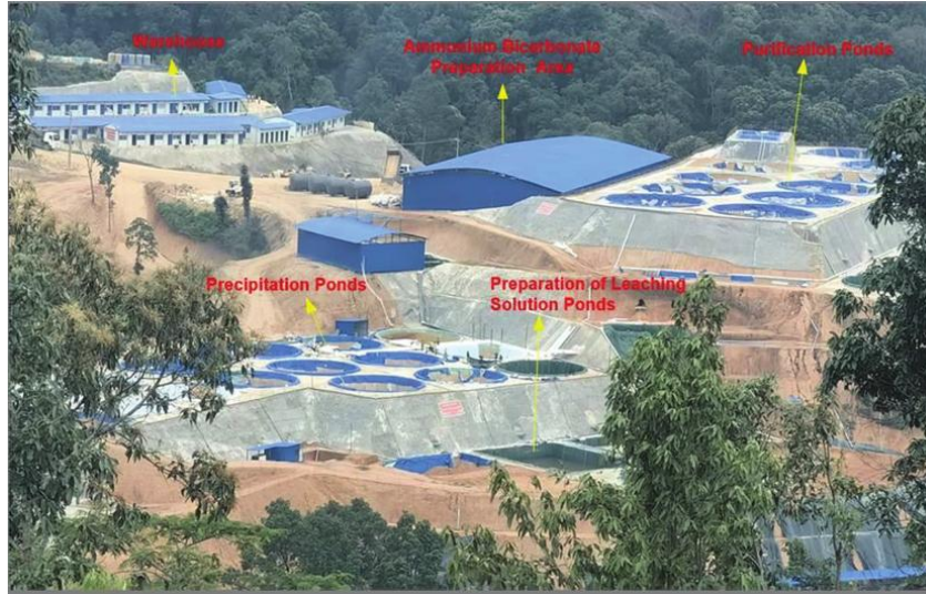
Figure 13-2: General View of the Hydrometallurgical Plant
