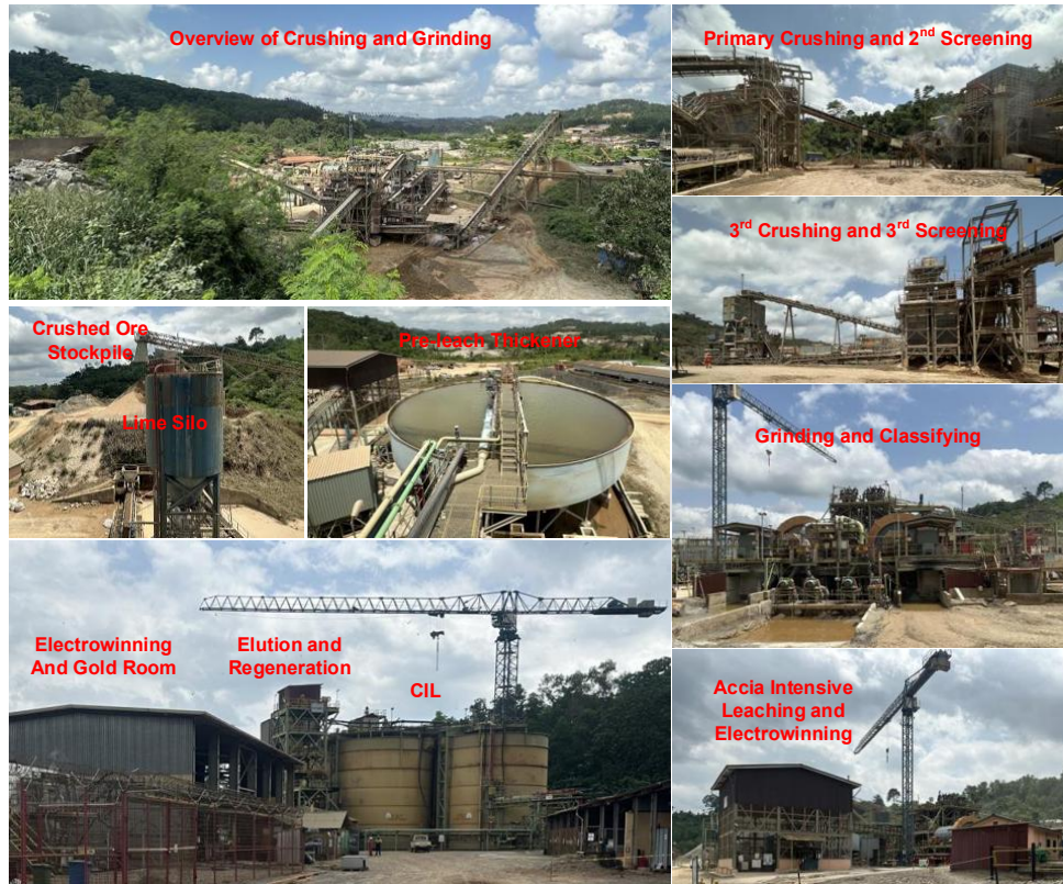
Figure 13-2: Photo of Wassa Processing Plant
