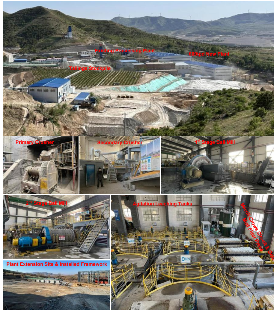
Figure 11-2: Site Photos of Jilong Processing Plant
