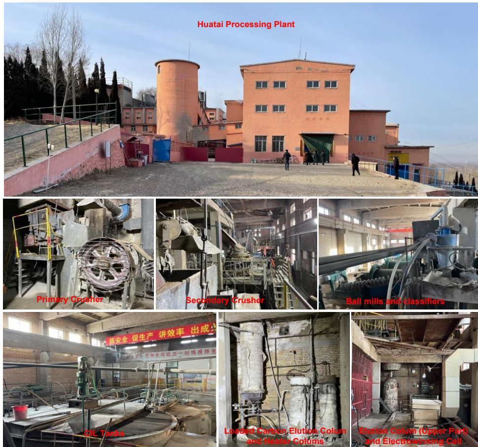
Figure 11-6: Site Photos of Huatai Processing Plant
