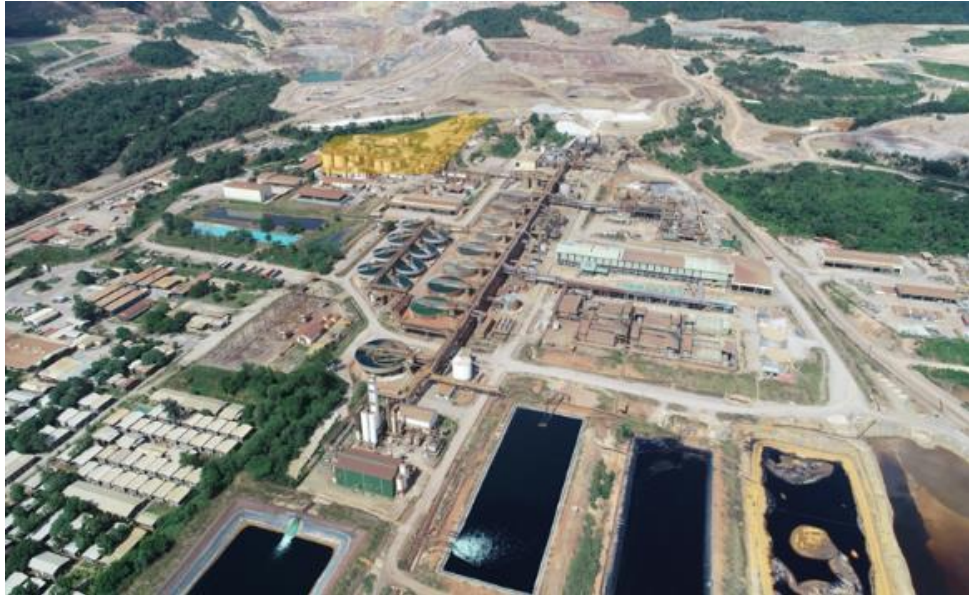
Figure 13-1: Sepon Gold Plant and Copper Plant Complex
