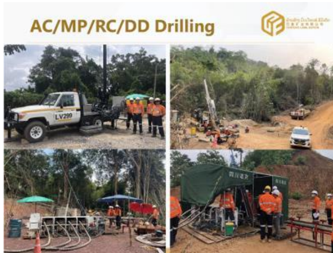
Figure 7-5: Drill rigs used in the exploration in Sepon Project
