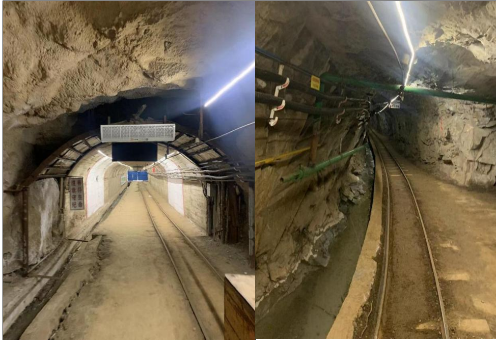
Figure 10-20: Photos of Access of Adit and Drift on Level 3 at Dongfeng Mine
