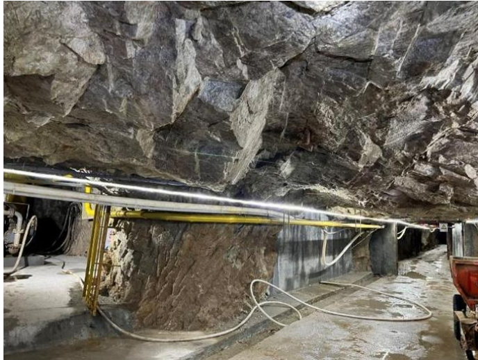
Figure 10-12: Level 7 in Zone 2 (-136m asl)
