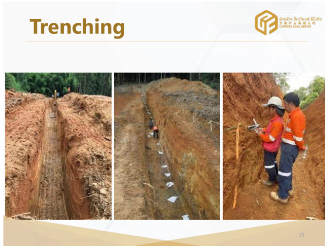
Figure 7-4: Trenches used in the exploration in Sepon Project
