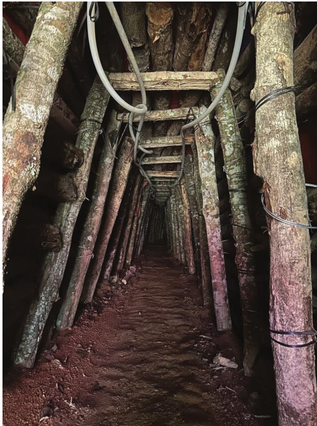
Figure 12-7: Main PLS Collection Tunnel in Construction
