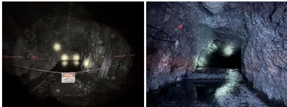
Figure 11-8 DSE UG Underground Site Visiting Photos
