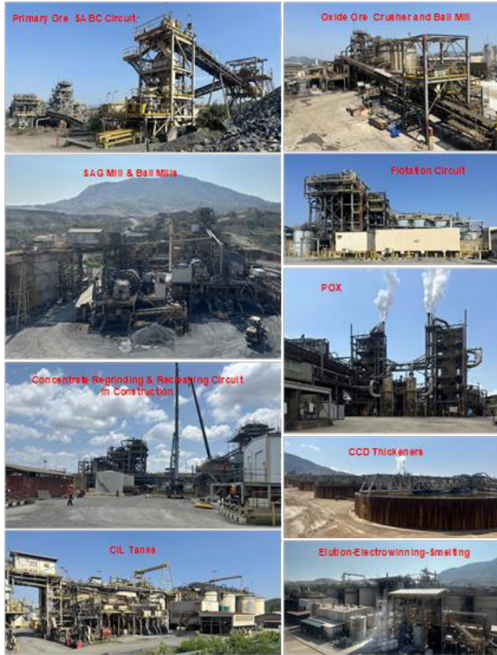
Figure 13-3: Facilities of Sepon Gold Plant
