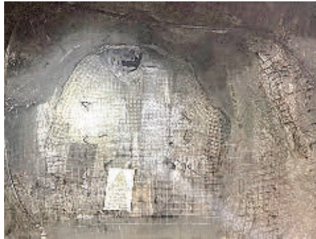
Figure 8-8: A Backfilled Heading
