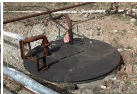
Buried elevated water tank, 800 m 3
