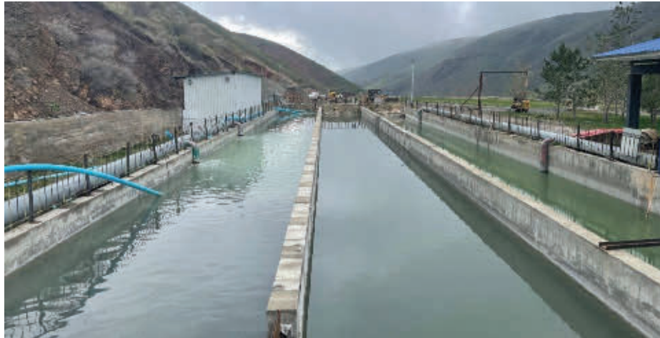
Figure 8-11: Sediment Pool for Mining Water Supply
