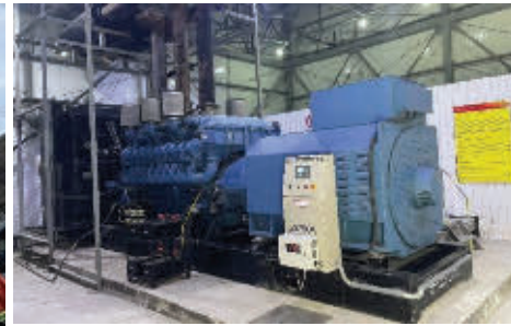
Standby diesel generator
