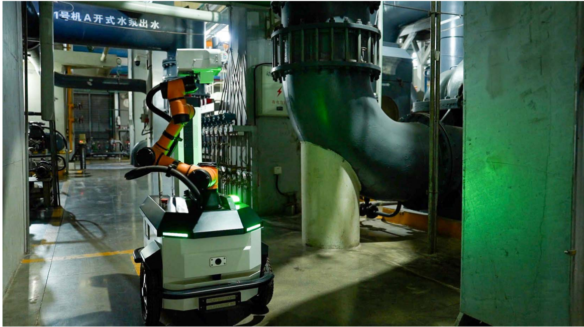
Inspecting the facility
