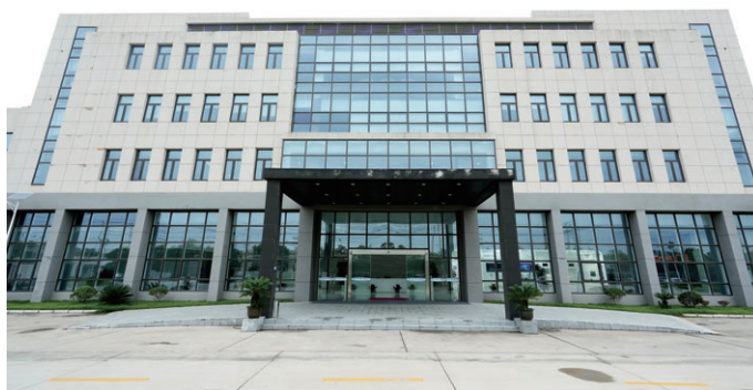
The image above shows the main building of our Dongtai facility.
