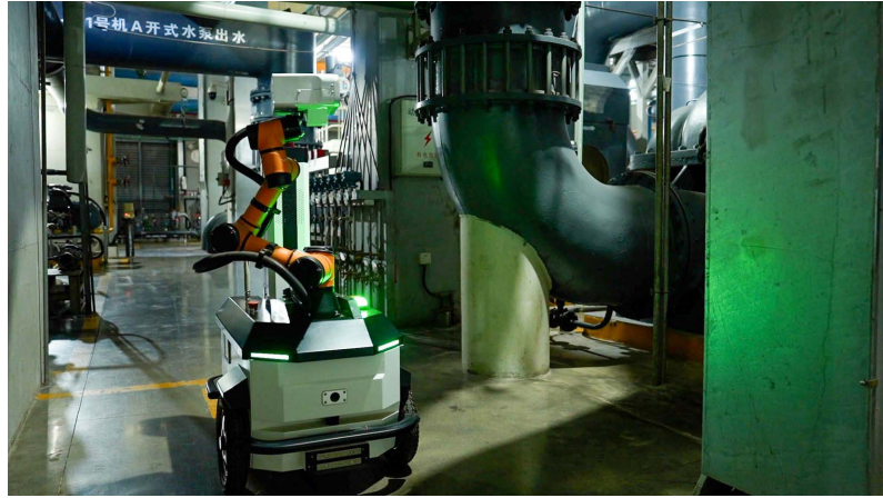
Inspecting the facility
