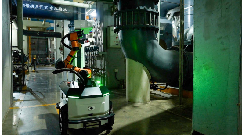
Inspecting the facility
