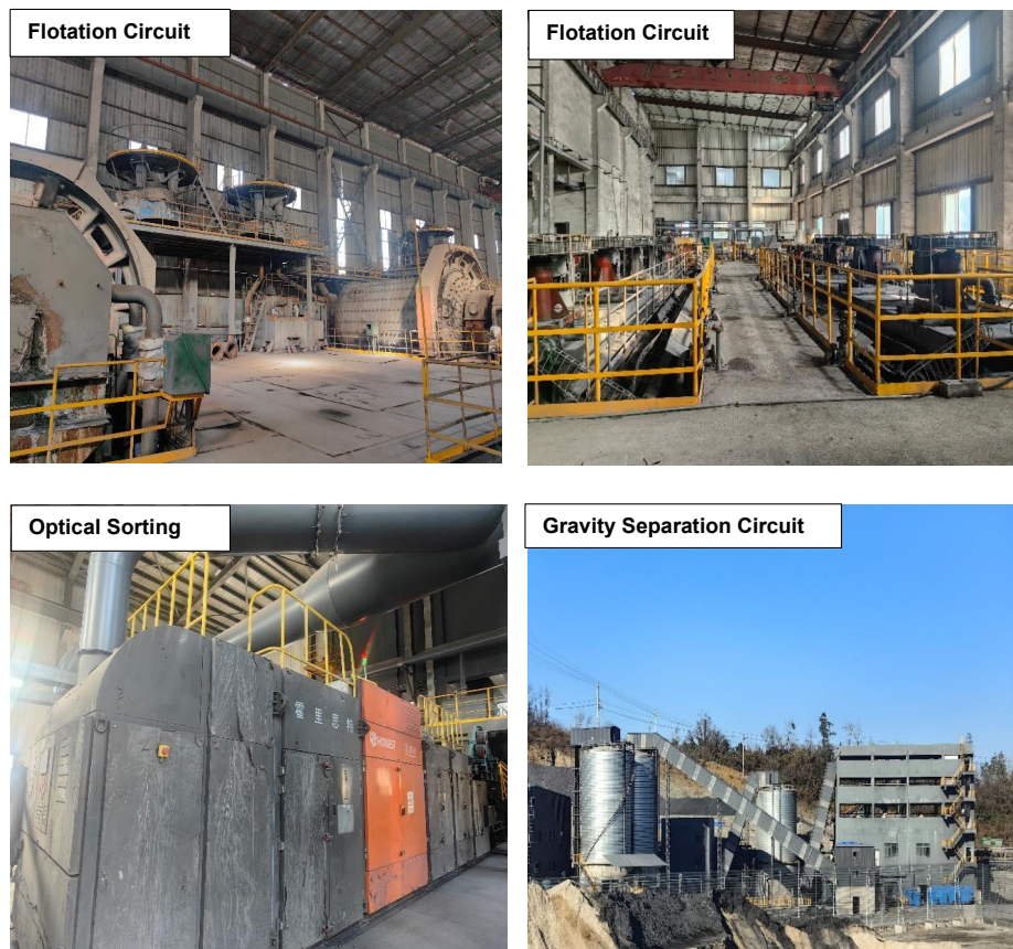
Figure 12-3: Selected Views of the Processing Facility.
