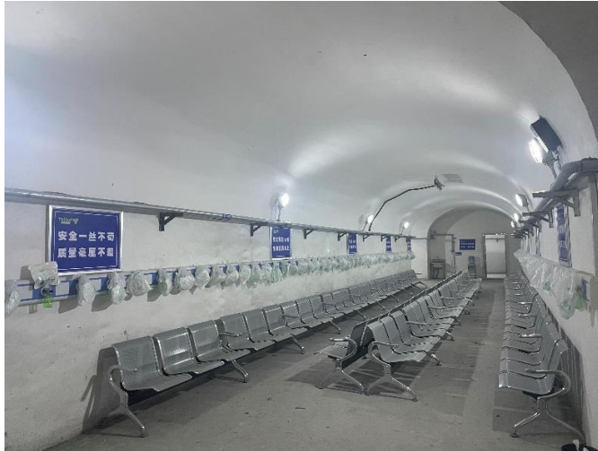
Figure 11-11: Emergency Refuge System
