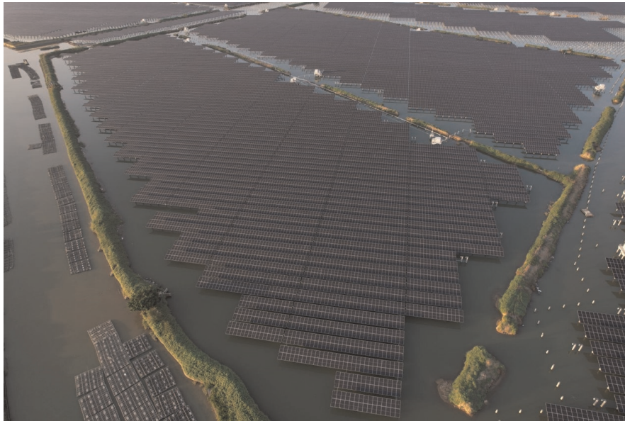
An offshore PV power project (海上光伏項目) in respect of which we have provided EPC services
