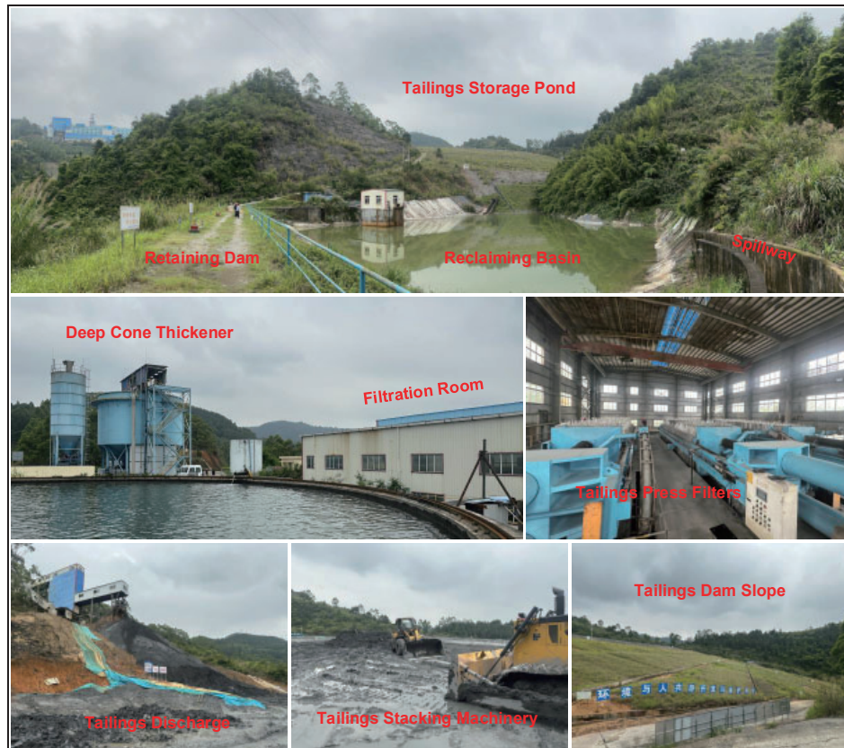
Figure 18.2: Photos of Tailings Storage Facility
