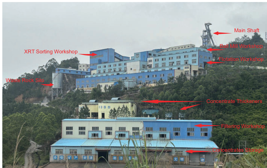
Figure 17.1: Photo of GC Processing Plant
