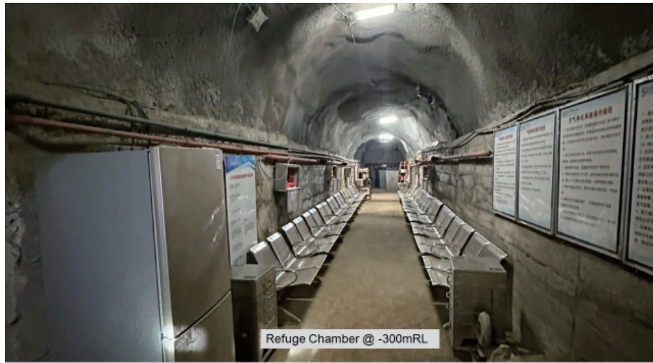
Figure 16.11: Permanent Refuge Station at -300ASL
