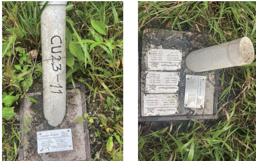
Figure 12.2: Condor Project Drillhole Sealing Mark
