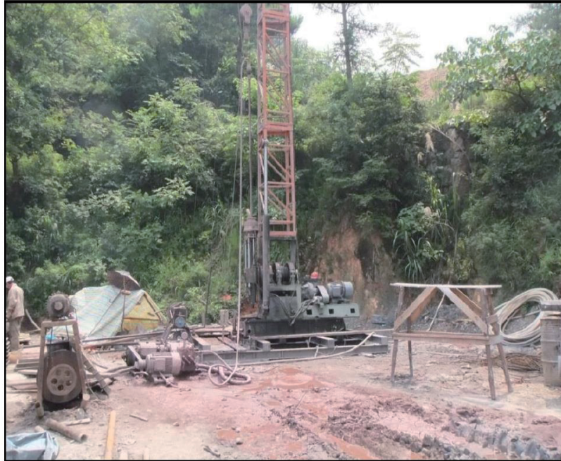
Figure 10.2: Drill Rig XY-42T at Hole ZK2110
