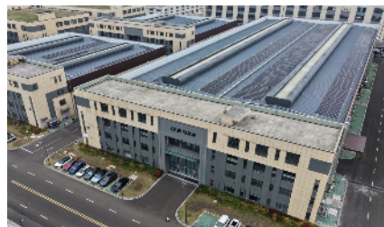
Ningbo Production Base
