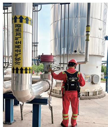
Performing leak detection on petrochemical facilities
