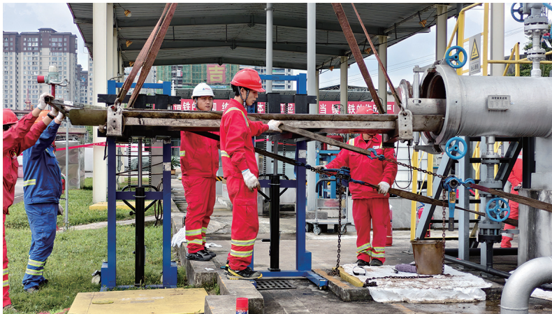
Performing magnetic flux leakage in-line inspection on pipeline launcher
