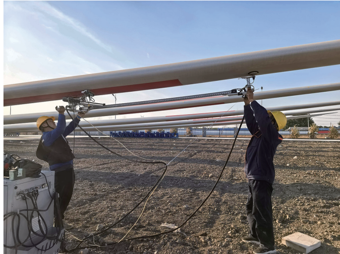
Performing pre-installation NDT for wind turbine blades
