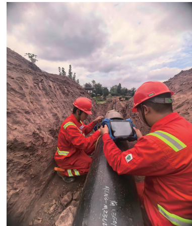
Performing on-site NDT on pipelines
