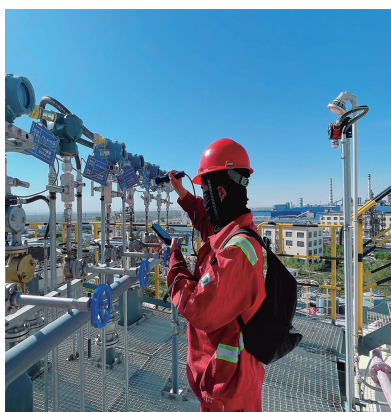
Performing leak detection on LNG facilities
