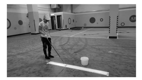
Depending on specific characteristics of the site and our customers' demands, we may be required to conduct screeding work and anti-skid surfacing work (for ramp surfaces) as part of our car park flooring procedures.
