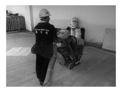
(iii) Surface preparation – repairing surface cracks
