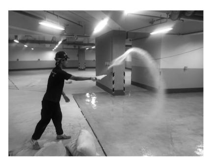
(vii) Removing excess quartz sand from the primer
