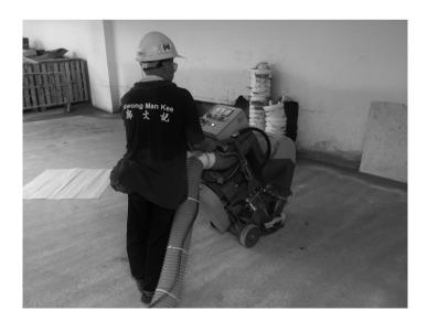
(iii) Surface preparation – repairing surface cracks
