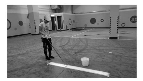
Depending on specific characteristics of the site and our customers' demands, we may be required to conduct screeding work and anti-skid surfacing work (for ramp surfaces) as part of our car park flooring procedures.
