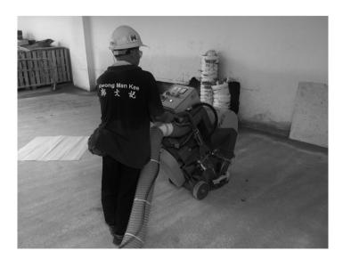
(iii) Surface preparation – repairing surface cracks
