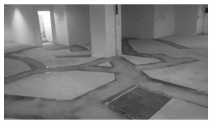
(iv) Surface preparation – substrate defects remedial work
