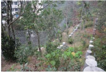
*Installation of debris flow protection rigid barriers*
