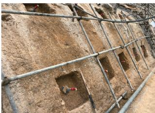
*Drilling and installation of soil nails*
