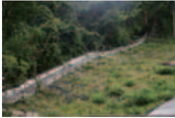
Construction of concrete maintenance stairway/access
