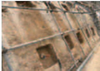
Drilling and installation of soil nails
