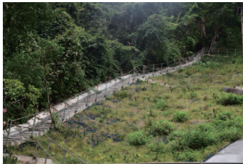
Construction of concrete maintenance stairway/access
