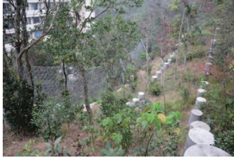
Installation of debris flow protection rigid barriers
