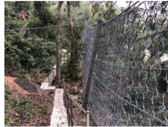
Construction of flexible barrier system
