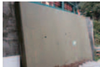
Construction of retaining walls
