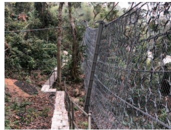
Construction of flexible barrier system
