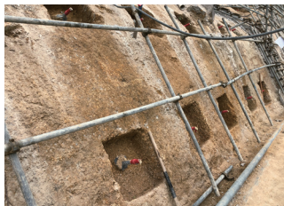
Drilling and installation of soil nails
