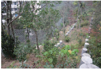
Installation of debris flow protection rigid barriers
