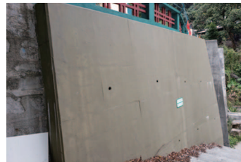
Construction of retaining walls
