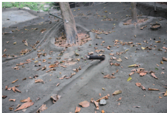
Installation of raking drains
