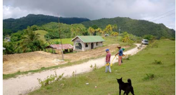
Tree planting along the access road participated by the CIMP personnel during their vacant time.
