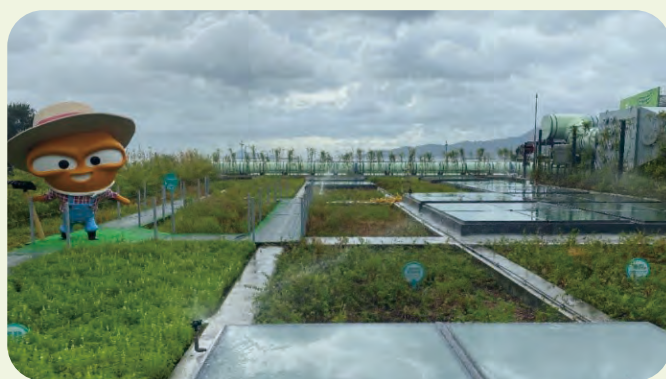
(Photo credit: Main Contractor) 圖片來源：承建商
