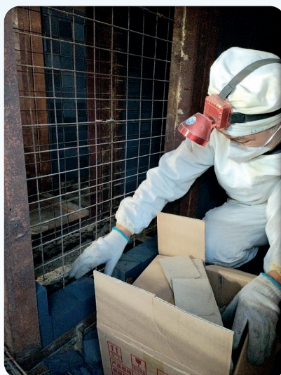
Figure 1 The activated carbon of the waste gas treatment equipment is replaced regularly every year at the Beijing production base
