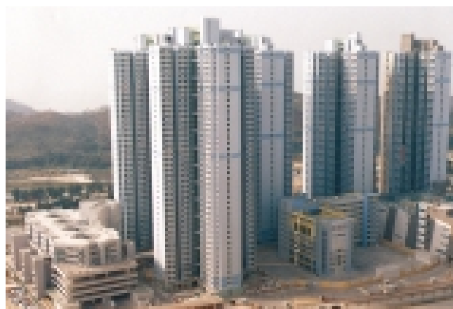
Public housing estate at Tin Shui Wai Area 105, Phase 1
