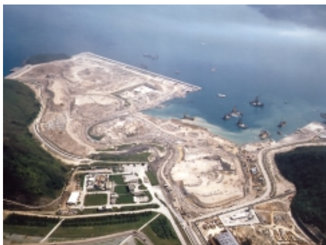
Construction of Seawalls and Reclamation at Tseung Kwan O Port Development at Area 137, Stage 2
