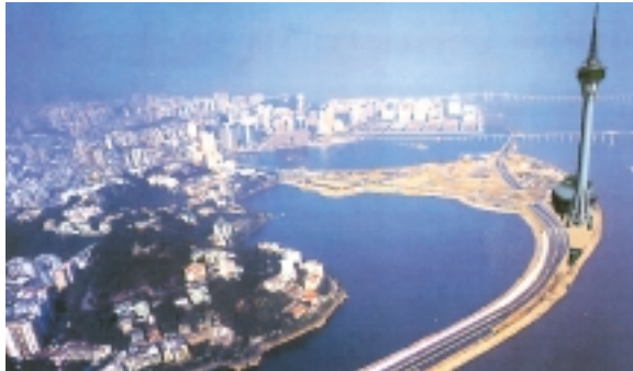
Lift and Escalator, Mechanical, Electrical and Fire Protection Installation for Macau Tower Entertainment Centre
