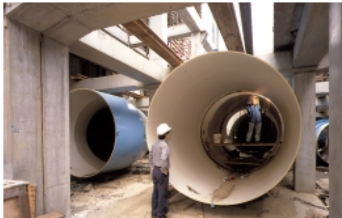
Pipe installation at Tai Po Water Treatment Works and Pumping Station
