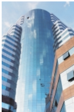
Harbour Ring Huang Pu Centre, Shanghai
