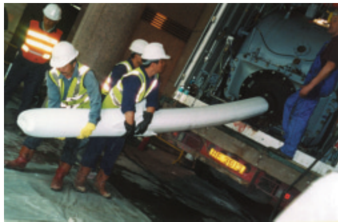
Repair of Underground Air Conditioning Cooling Intake Pipes by Process Phoenix for Wing On House, Central
