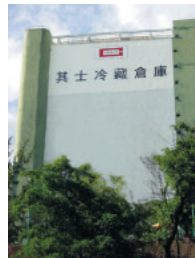
An eighteen-storey warehouse located at Kwai Chung
