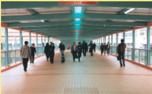
旺角行人天橋 1 期 Mongkok pedestrian overpass Phase I
