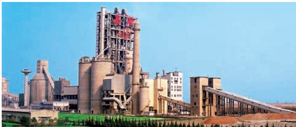
Outlook of the Group's production facility 集團生產基地外貌
