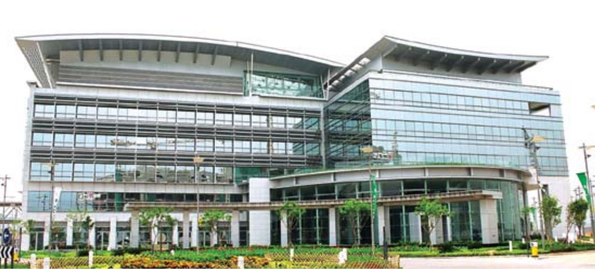
Science Park, Buildings 1 and 2 科學園1及2號樓
