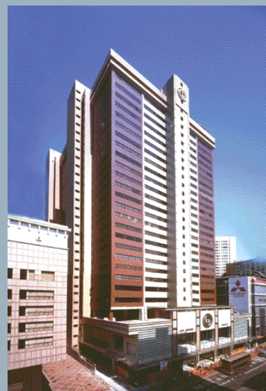
荃灣中染大廈之維修、改建及加建工程 Renovation, Alteration and Addition Works for The CDW Building in Tsuen Wan
