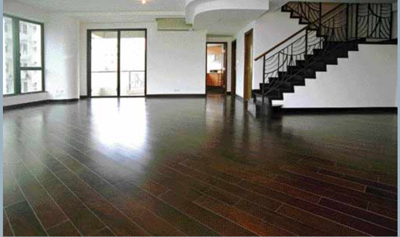
為肇輝臺供應及安裝木地板 Supply & Installation of Timber Flooring for Shiu Fai Terrace
