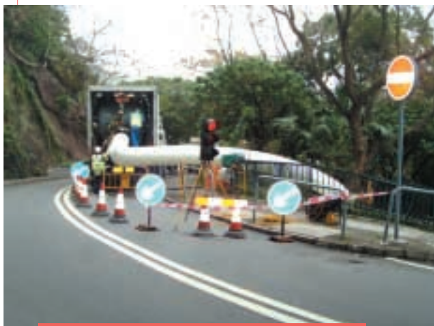
Installation of 600mm diameter Phoenix Pipe Liner at Repulse Bay
