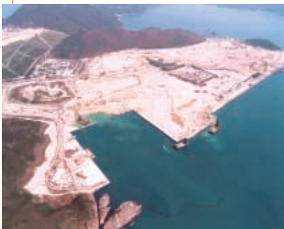
Construction of Seawalls and Reclamation at Tseung Kwan O Port Development
