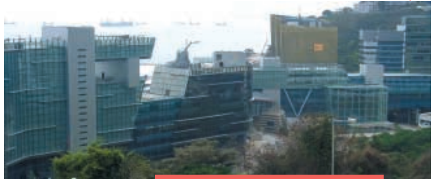
Installation of aluminium engineering works at Cyberport Development
