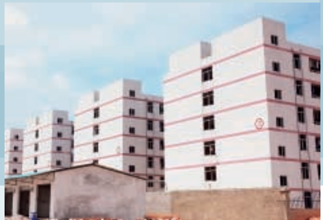
■ 員工宿舍 Staff Dormitory
