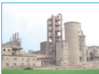
山東水泥位於山東之廠房 Factory buildings of Shandong SAC in Shandong
