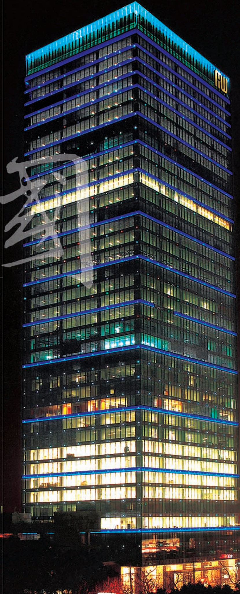
Shanghai K. Wah Centre, Huaihai Zhong Road, Shanghai
