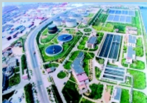
Qingdao Haibohe Waste Water Treatment Plant 青島海泊河污水處理廠
