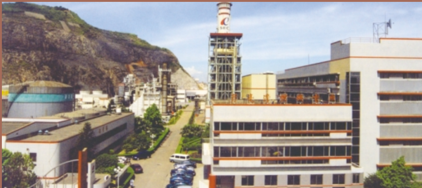
Yueliangwan Power Plant of Shenzhen Mawan Power Company 深圳媽灣電力公司之月亮灣電廠
