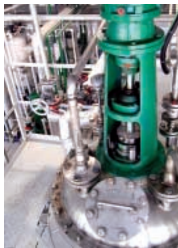
The Zhuhai Plant Workshop
