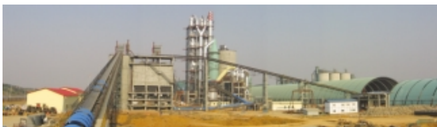
已建設完成位於廣西貴港的日產5,000噸新型乾法水泥熟料新生產線 Our newly completed 5,000 tonnes per day NSP clinker production line in Guigang, Guangxi
