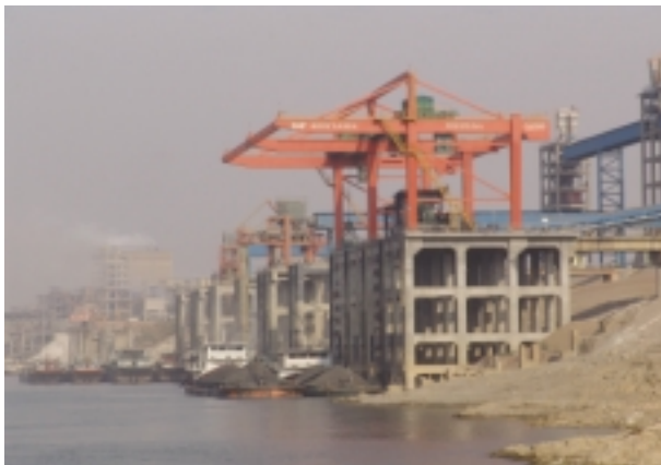
本集團位於廣西平南水泥生產基地的附設碼頭 The Group's pier attached to the cement production site at Pingnan, Guangxi
