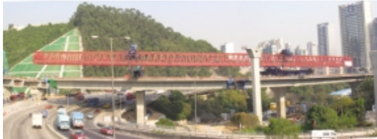
八號幹線(荔枝角道) – 本集團製造的預製混凝土高架橋段樑 Route 8 (Lai Chi Kok Viaduct) – precast concrete bridge viaduct produced by the Group
