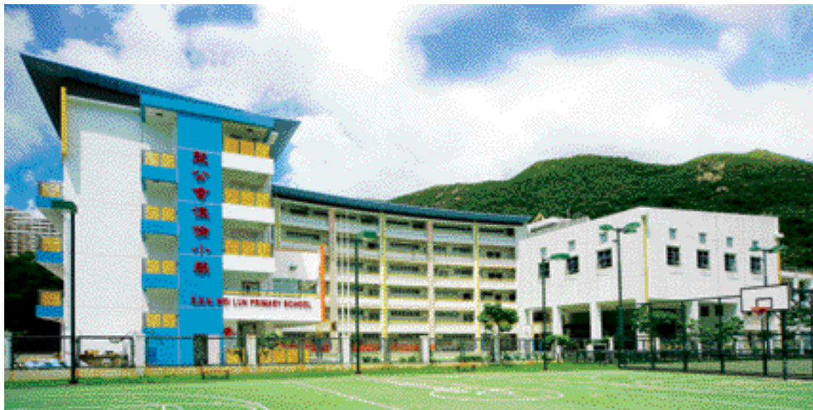
▲ School improvement work for S.K.H. Wei Lun Primary School 聖公會偉倫小學之改建工程
