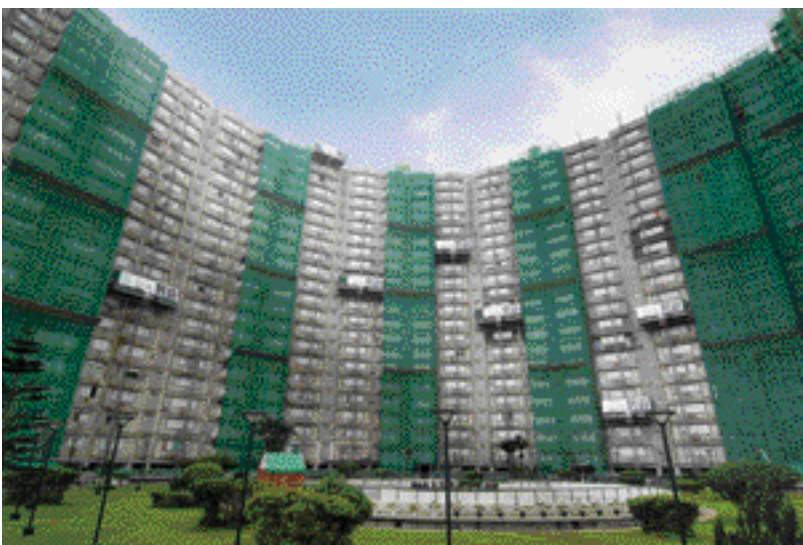
◀ Renovation works for Villa Monte Rosa 玫瑰新村維修工程
