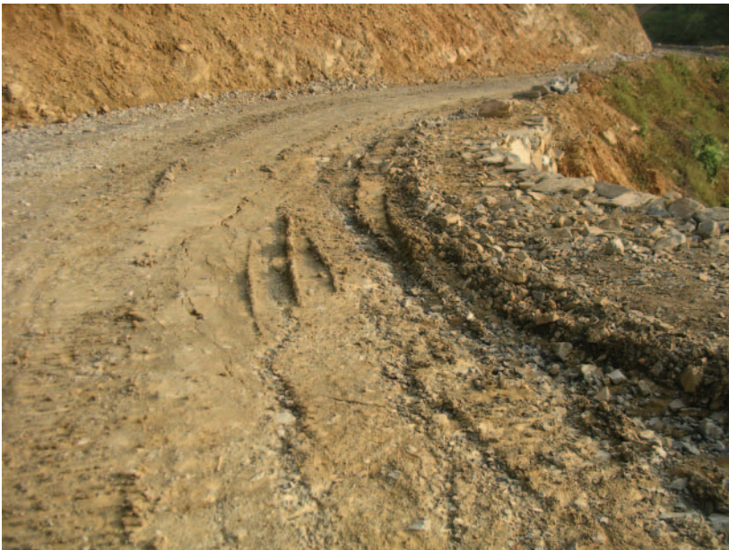
Figure 5-15: Incipient Failure of Retaining Structure on CIL Storage Facility Access Road, 15 October 2006
