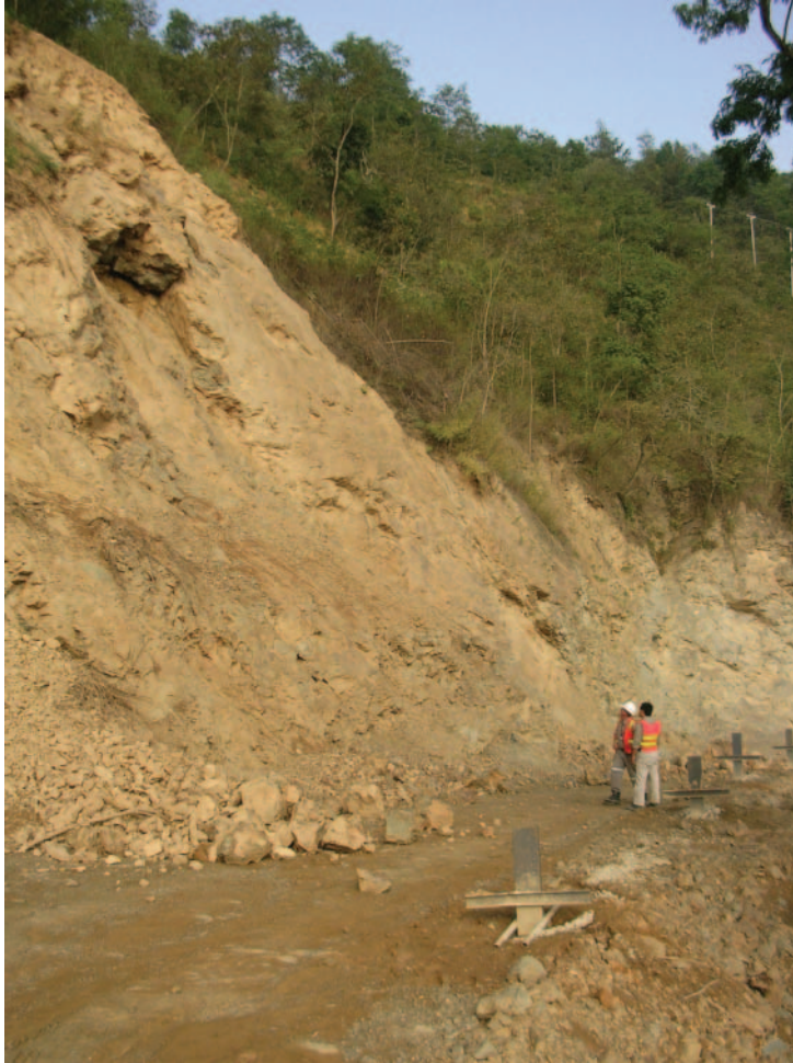
Figure 5-14: Recent Failure on Access Road to CIL Storage Facility, 15 October 2006
