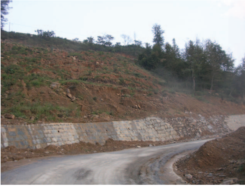
Figure 5-12: Unstable Slope on Main Access Road to Plant, 15 October 2006
