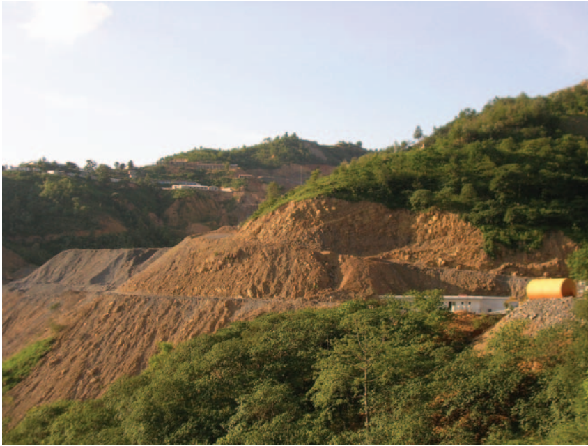
Figure 5-6: Photograph Showing Main Decline Portal Area, 15 October 2006
