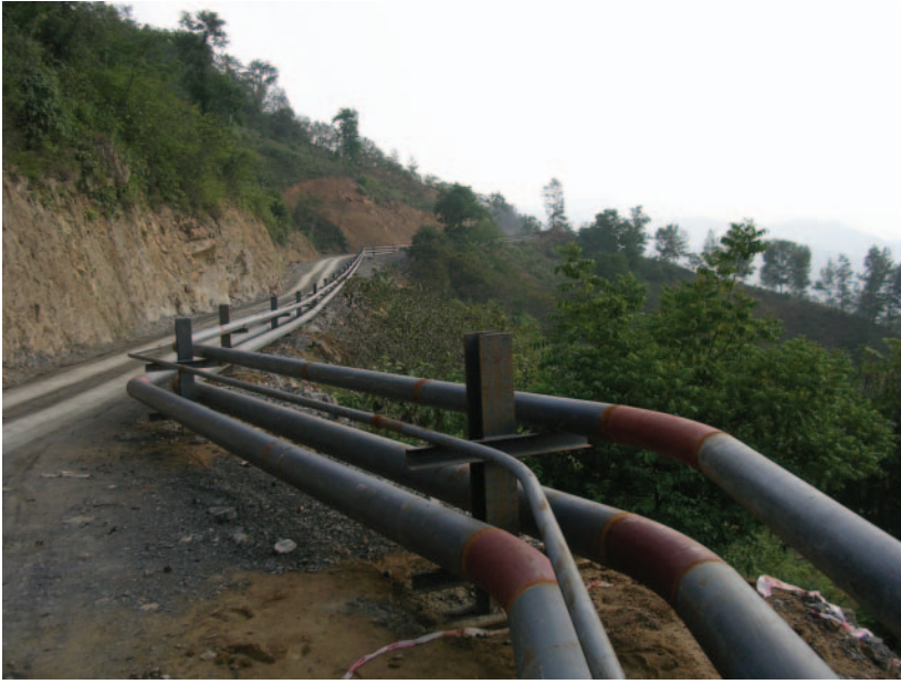
Figure 5-13: Access Road to Tailings Storage Areas, 15 October 2006
