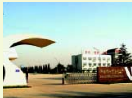
Jinan No. 2 Waste Water Treatment Plant 濟南市水質淨化二廠
