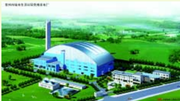
Changzhou Waste-to-energy Plant 常州垃圾焚燒發電廠
