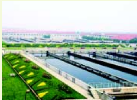
Jinan Waste Water Treatment Plant 濟南污水處理廠
