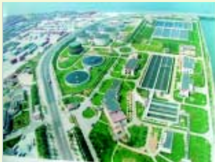
Qingdao Haibohe Waste Water Treatment Plant 青島海泊河污水處理廠
