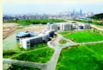
Suzhou Waste-to-energy Plant (Dormitory building) 蘇州垃圾焚燒發電廠（生活樓）
