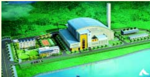
Jiangyin Waste-to-energy Plant 江陰垃圾焚燒發電廠
